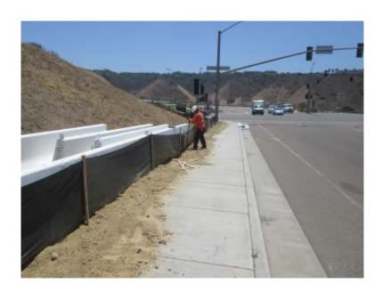
**Photo 2:** BMP's consisting of silt fence were installed along the perimeter of the project site in accordance with the SWPPP and MM-HYD-1.
