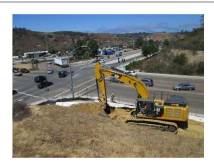
**Photo 1:** Construction crews completing ground disturbance activities within the approved work limits to establish an access road along the perimeter of the project site.
