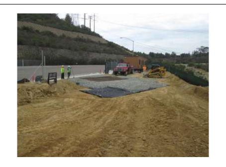
**Photo 3:** Trac-out control measures have been installed at the construction site entrance in accordance with the SWPPP and MM-HYD-1. Trac-out controls consisted of rattle plates and a rock apron in order to minimize trac-out onto paved public roads.
